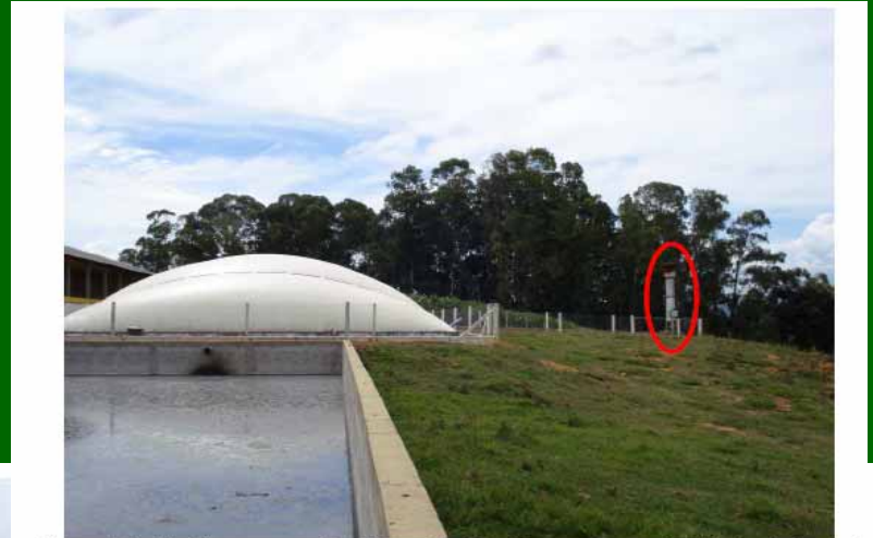
Figure A.4. – Biodigester system in white and enclosed flare system on the right in the farm of Sergio Tassi.
